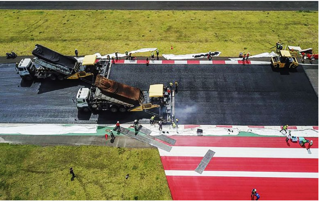
Photos: Resurfacing of the Mandalika Circuit main track using Stone Mastic Asphalt (SMA) over a stretch of 1.2 km from Turn 17 to Turn 5.
