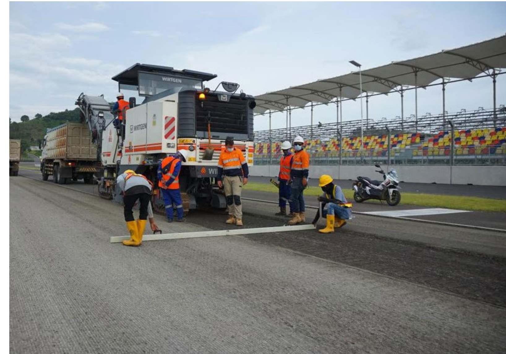
Photo: Re-paving of the Mandalika Circuit ahead of the MotoGP 2022 event. The re-paving was required after sections of the track surface peeled during the pre-season test on 11-13 February 2022.
