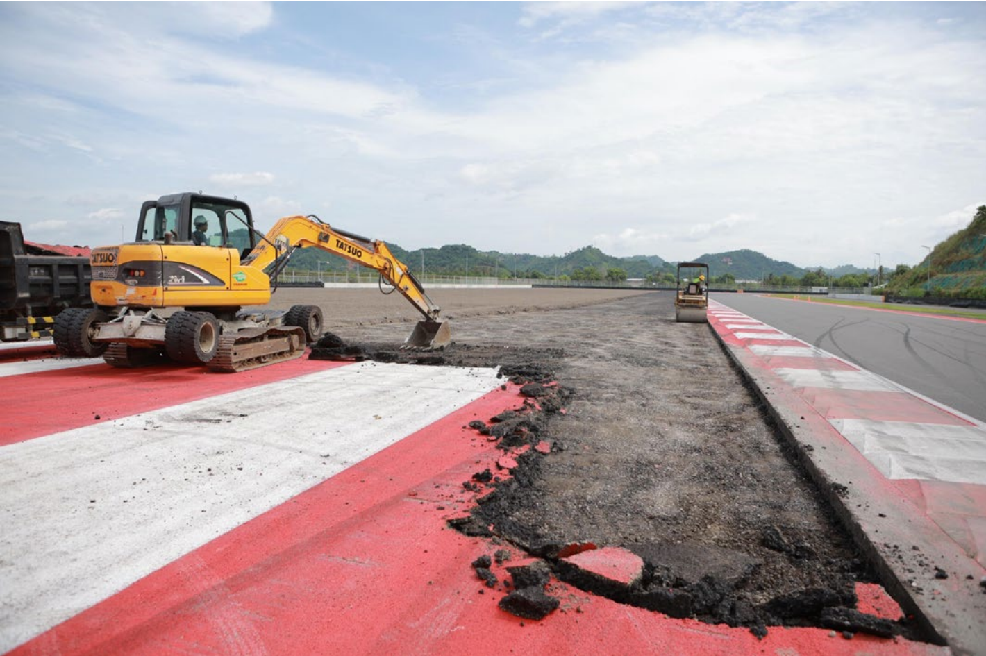
Photo: FIA homologation process for Mandalika International Circuit involves a series of physical modifications carried out since 11 March 2025. Modifications include, among others, asphalt removal in run-off areas and addition of gravel traps at strategic points such as T1 Exit/T2 Entry, T5 Entry, T10 Entry, T10 Exit/T11 Entry, and T13 Entry.
